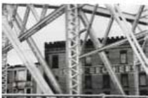
Mill Street Bridge Shawn Dougherty Pulaski, Pennsylvania
